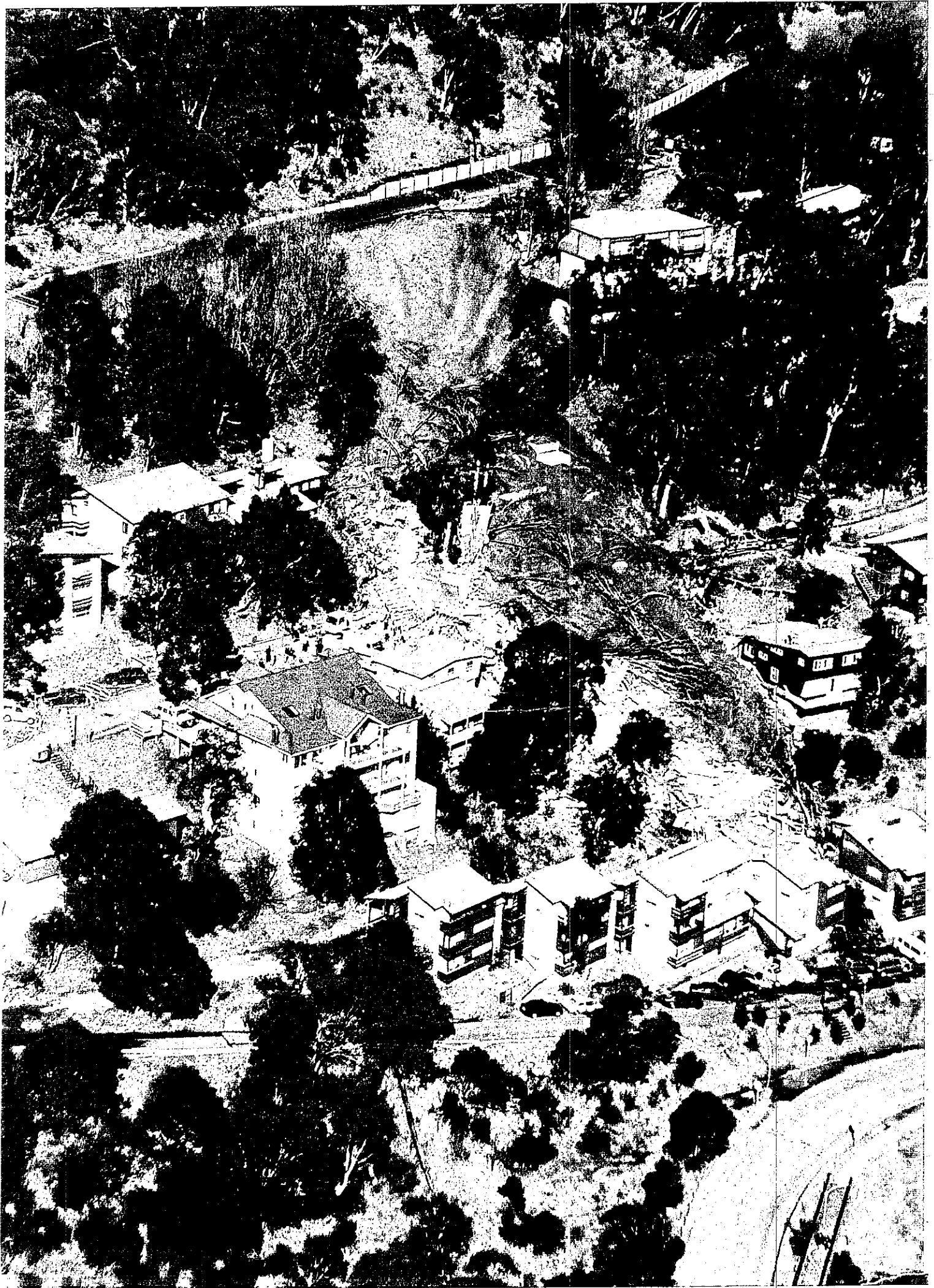
Fig 2. Aerial View of the Landslide
