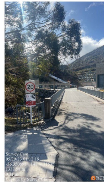
Reference 8 on Map - Murrumbidgee Power Station
